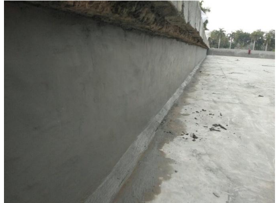
Grout coming out of joints in the floor while pressure grouting
