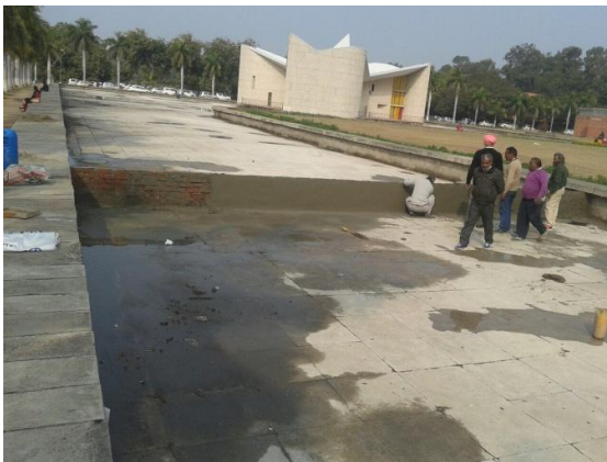
Construction of new wall to enclose 500sq mtr area gauge to measure water level
