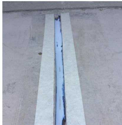
QS- 530 poured into the cut joints
