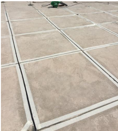
Masking of joint edges with tape
