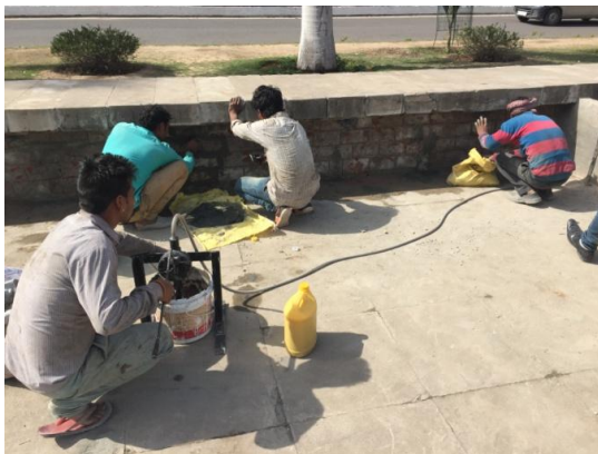
Pressure grouting being done with a manual pump spaces in the wall
