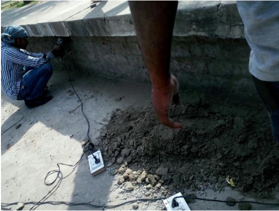
Removing plaster with mechanical means cutter
