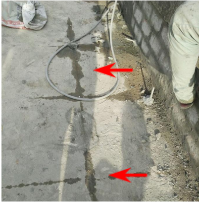
Grout coming out of joints in the floor while pressure grouting
