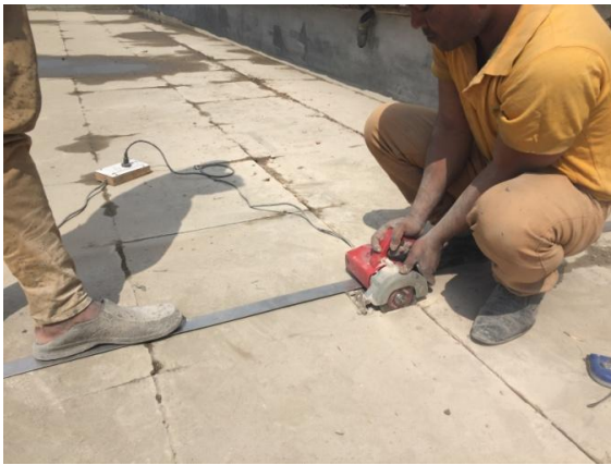
Cutting of floor joints
