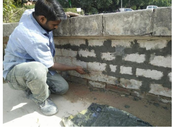
Sealing the joints with High
