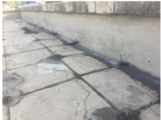
Grout coming out from the floor
