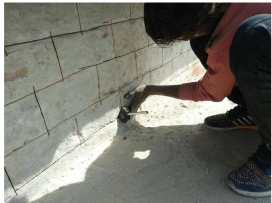
Inserting nipples into the holes
