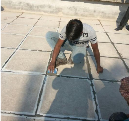
Sealing of joints with High Bond 40 mix into the holes.
