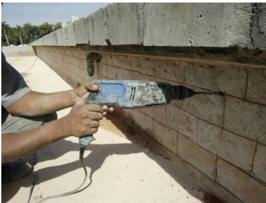
Removing plaster with mechanical means cutter
