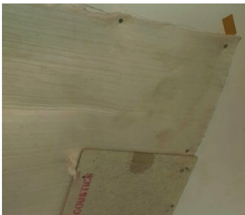
Acoustic Fleece as a base layer fixed on top of base layer
