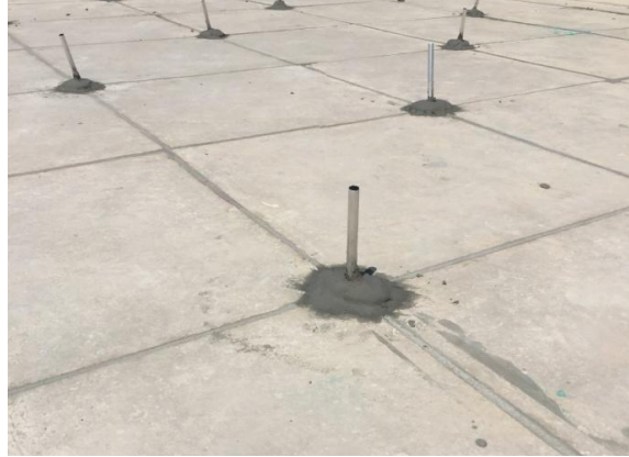
Inserting & fixing nipples 2" deep
