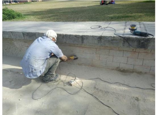
Cutting construction joints with
