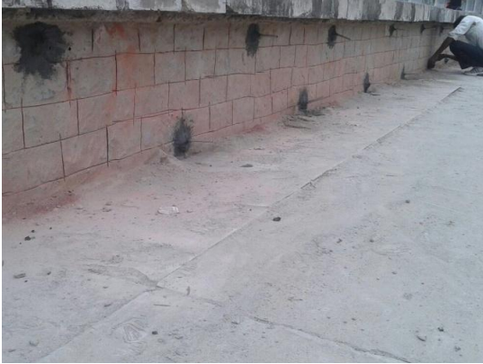
3ft spacing of the nipples covering 5sqft area each Bond 40 & cement
