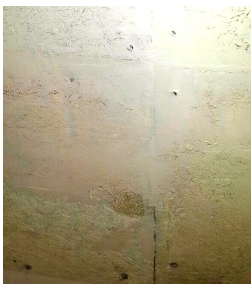
Joints flushed with Epoxy resin finished
