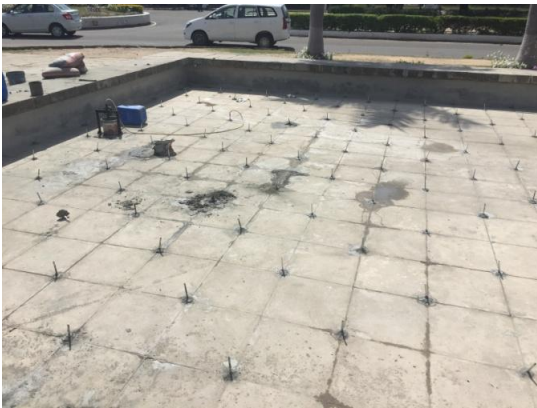
Sealing of joints with High Bond 40 mix into the holes.
