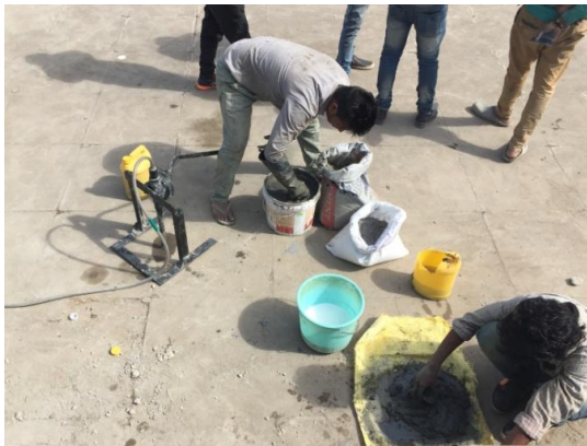
Mixing of compounds with cement pressure grouting
