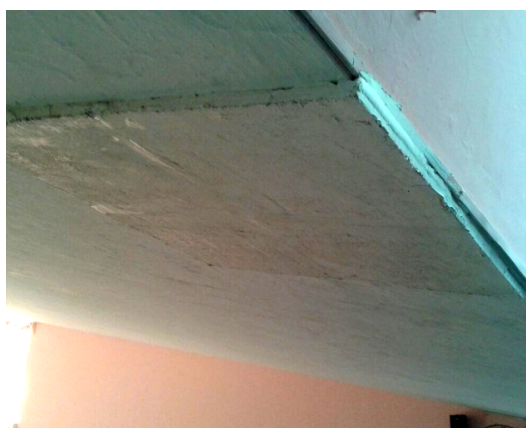
Rough edges and joints
