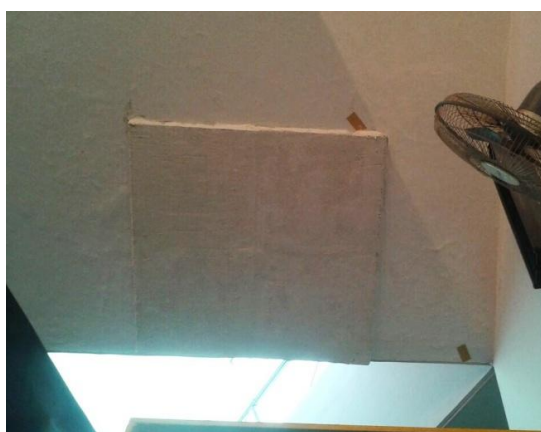
White cement putty base for top layer of paint with ceiling
